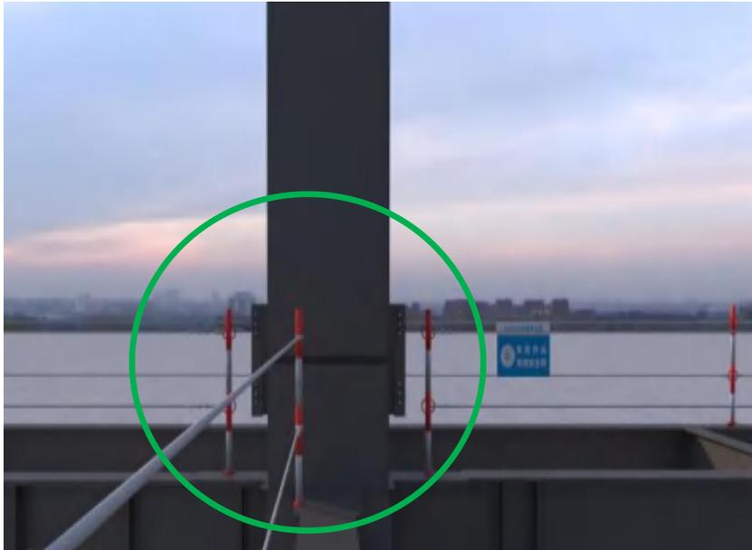
A photograph showing a construction site with a steel beam used as a horizontal passage. A green circle highlights the safety rope on the left side of the beam, which is continuous, indicating a correct safety practice. |
